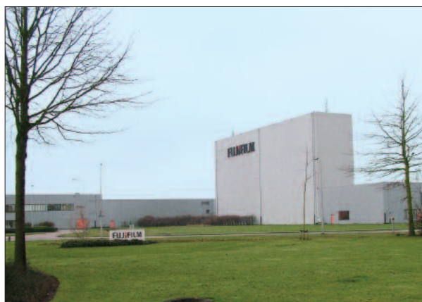
FUJIFILM Manufacturing Europe B.V. Plant
